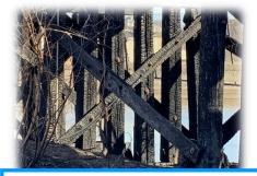
Severe Fire Damage to Bridge South Approach Requires Installation of New Support Piers and New Decking.
